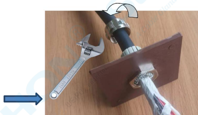
8) Tighten the compression nut and the main part by using a wrench. Refer to the torque listed in below table.
